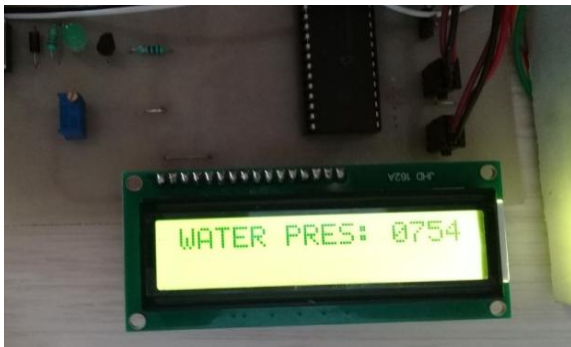
Fig.10: Displays water pressure reading
